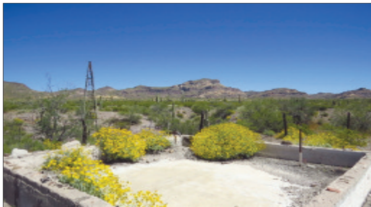
The windmill at Hummingbird Springs is broken and no longer pumps water into the tank, but there is still water in the bottom of the arroyo at the base of the old windmill.
