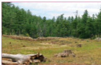
This is a breached dam on Schnebly Hill Road.
