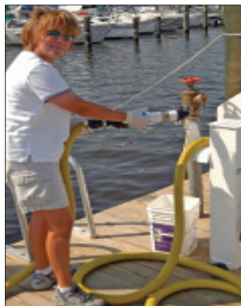
APPLY ASAP – A program funded by the taxes and fees paid by boaters can help pay for a boat pumpout facilities on your local waterway.
