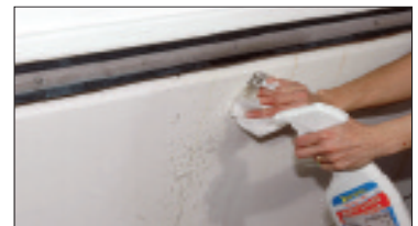
Remove Rust Stains
