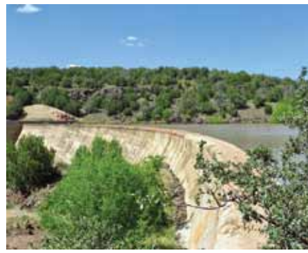
Ash Fork Stone Dam is at a lower elevation and is in the junipers.
