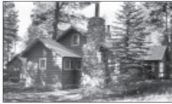
North Rim Ranger Residence
