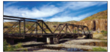
BRIDGE OVER — This is the bridge over the San Francisco River at Clifton.
