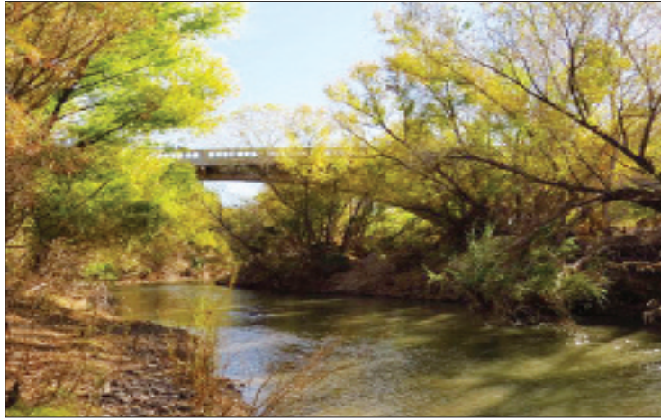
HOP IN HERE — This is a view of the Old Safford Bridge from the river where you put your boat in the water to start the float adventure. It is beautiful here!
