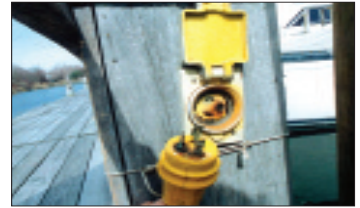
DANGER! — This shore power pedestal inlet and cable aren’t that far away from sparking a major boat fire.
