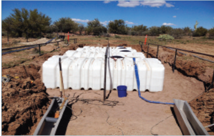
Tanks In Ground
