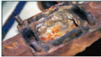
Corroded Exhaust Manifold
